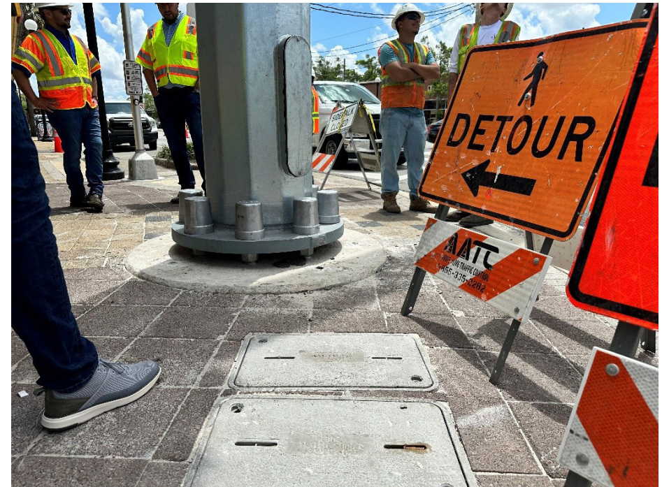
Figure 93: Example of a New Mast Arm and Foundation during Construction
