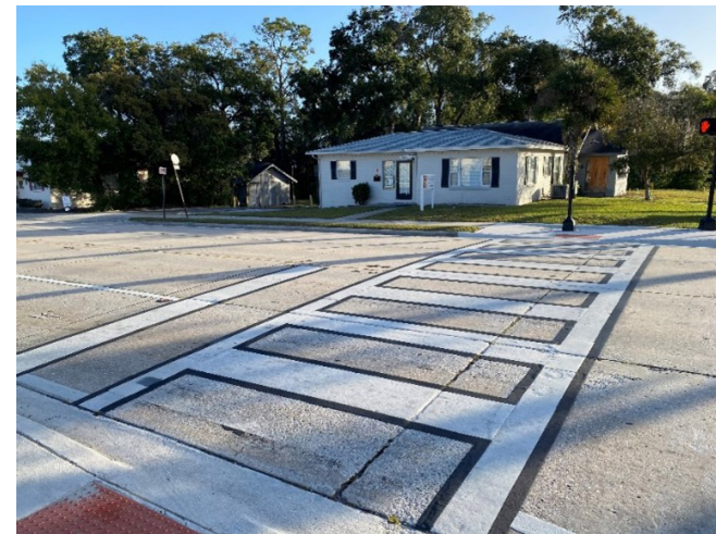
Figure 84: High-Contrast Black Outline Markings on Mills Ave
