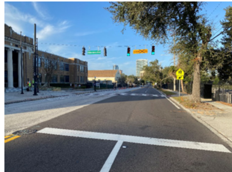
Figure 102: Pedestrian Traffic Control Signal on Robinson Street
