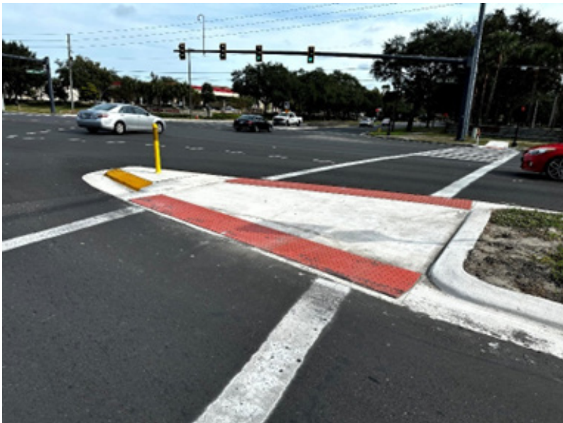
Figure 103: New Signalized Crosswalk and Concrete Refuge on SR 434
