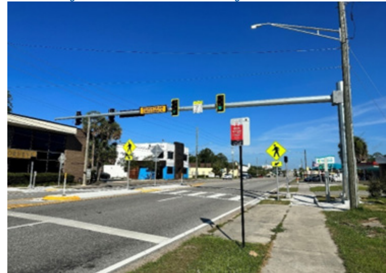
Figure 101: Midblock Pedestrian Signal in Jacksonville
