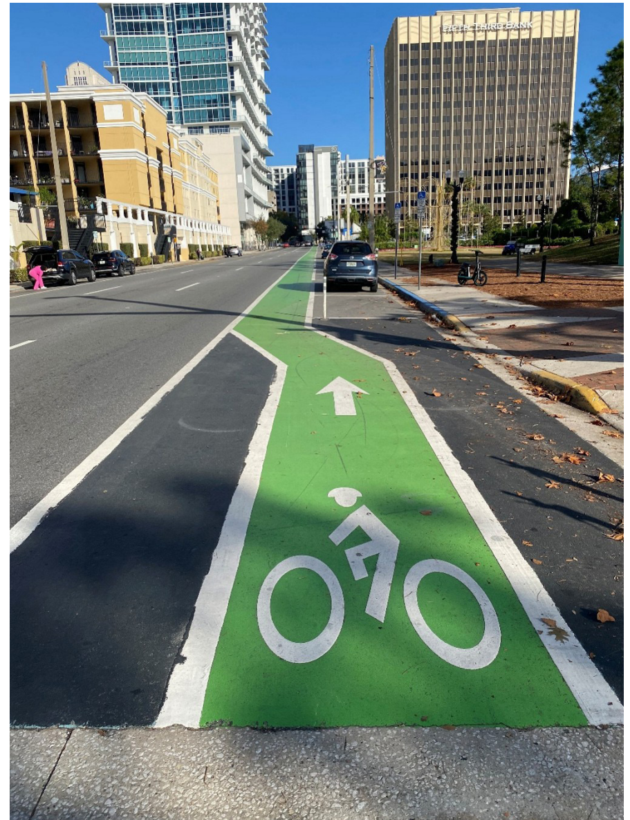
Figure 86: Solid Green-Colored Bicycle Pavement Markings on Rosalind Avenue
