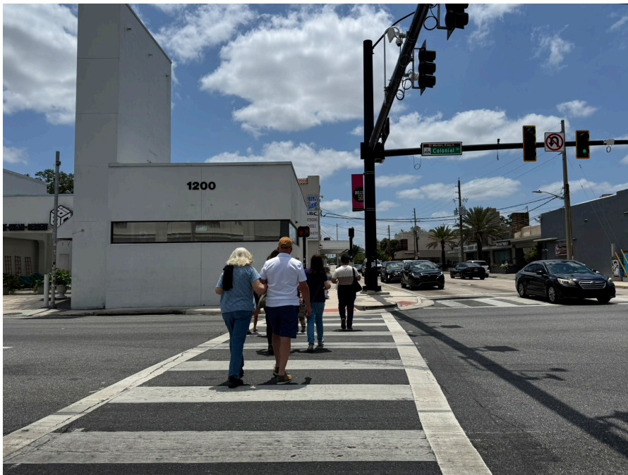
Figure 88: Special Emphasis Ladder Crosswalk on Colonial Drive
