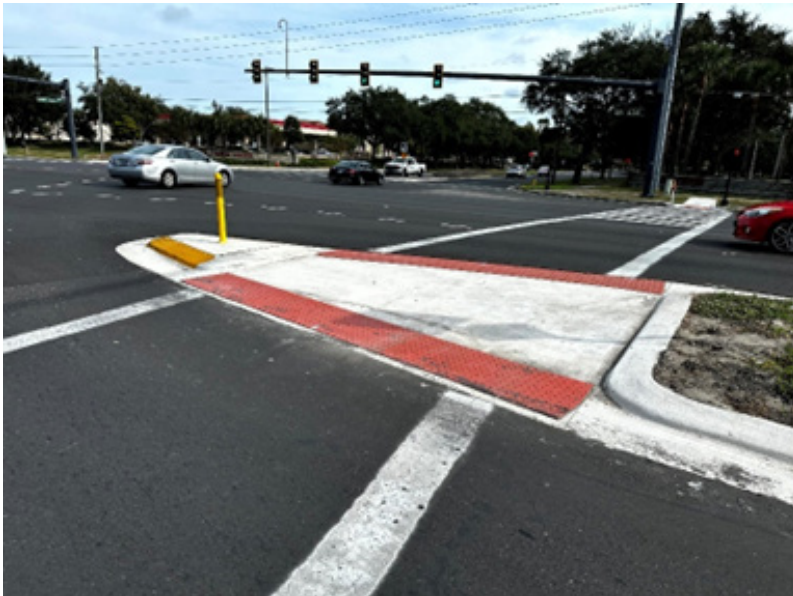
Figure 108: New Signalized Crosswalk and Concrete Refuge on SR 434
