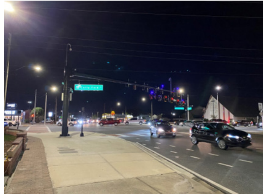
Figure 109: Intersection Lighting Enhancements on Curry Ford Road
