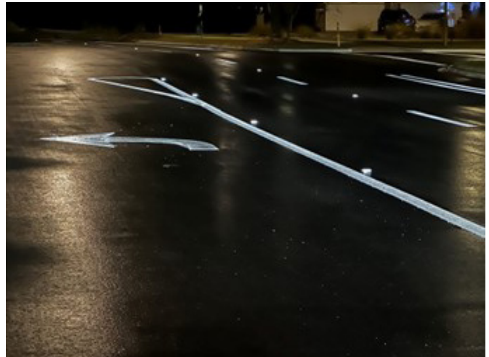
Figure 93: Photo of Raised Pavement Markers (RPMs) during Wet Nighttime Conditions
