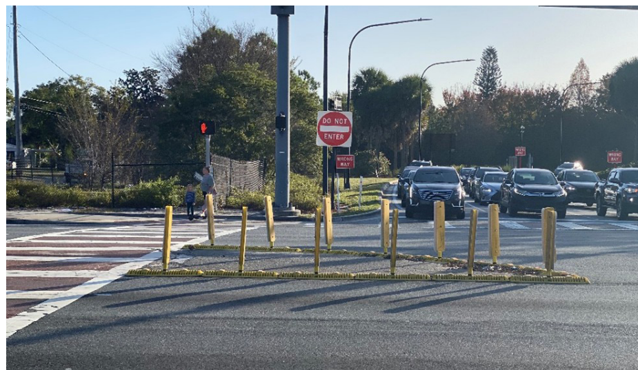
Figure 86: Photo of Curb Extension (Bulb-Out) on Rosalind Avenue
