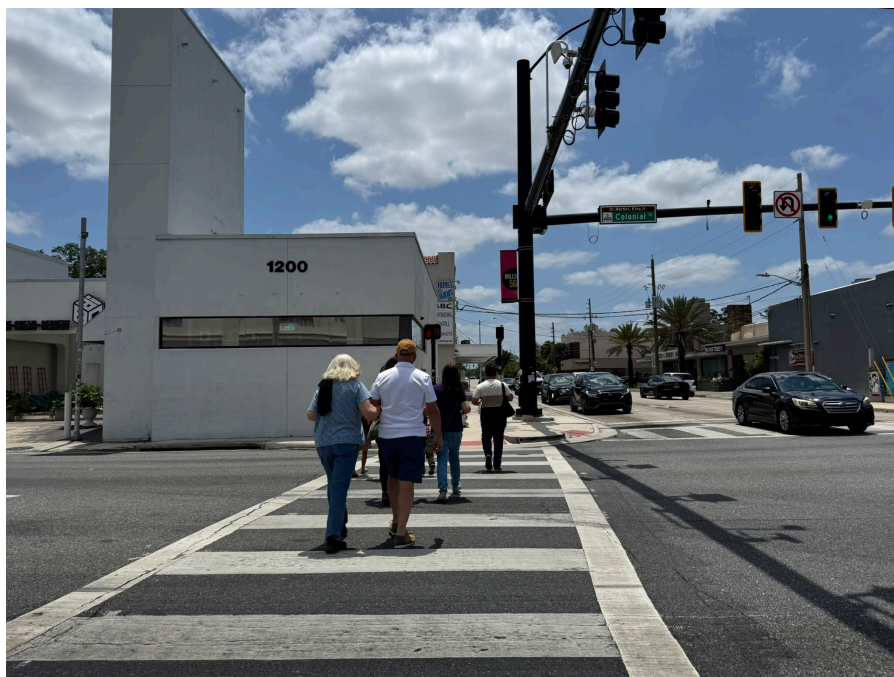
Figure 77: Special Emphasis Ladder Crosswalk on Colonial Drive
