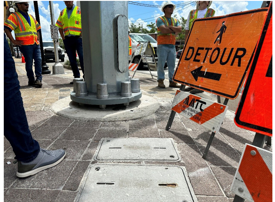
Figure 87: Example of a New Mast Arm and Foundation during Construction
