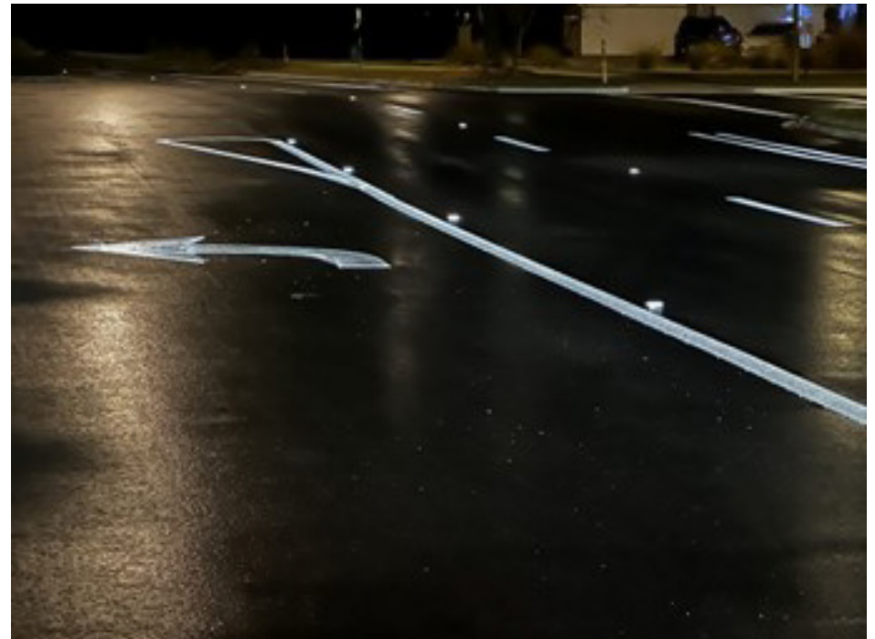
Figure 82: Photo of Raised Pavement Markers (RPMs) during Wet Nighttime Conditions
