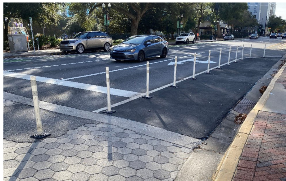
Figure 86: Photo of Curb Extension (Bulb-Out) on Rosalind Avenue
