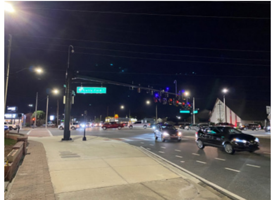
Figure 98: Intersection Lighting Enhancements on Curry Ford Road
