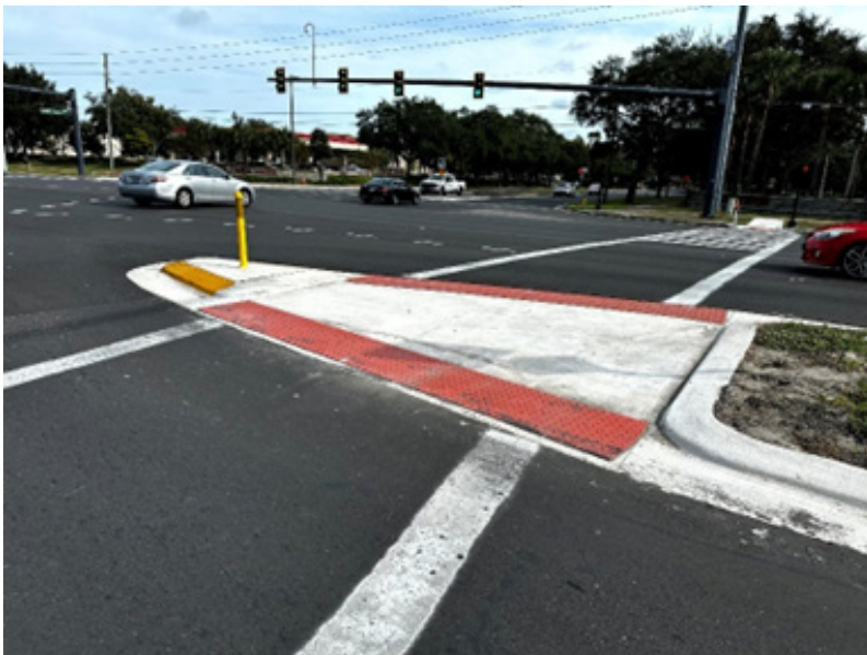
Figure 97: New Signalized Crosswalk and Concrete Refuge on SR 434
