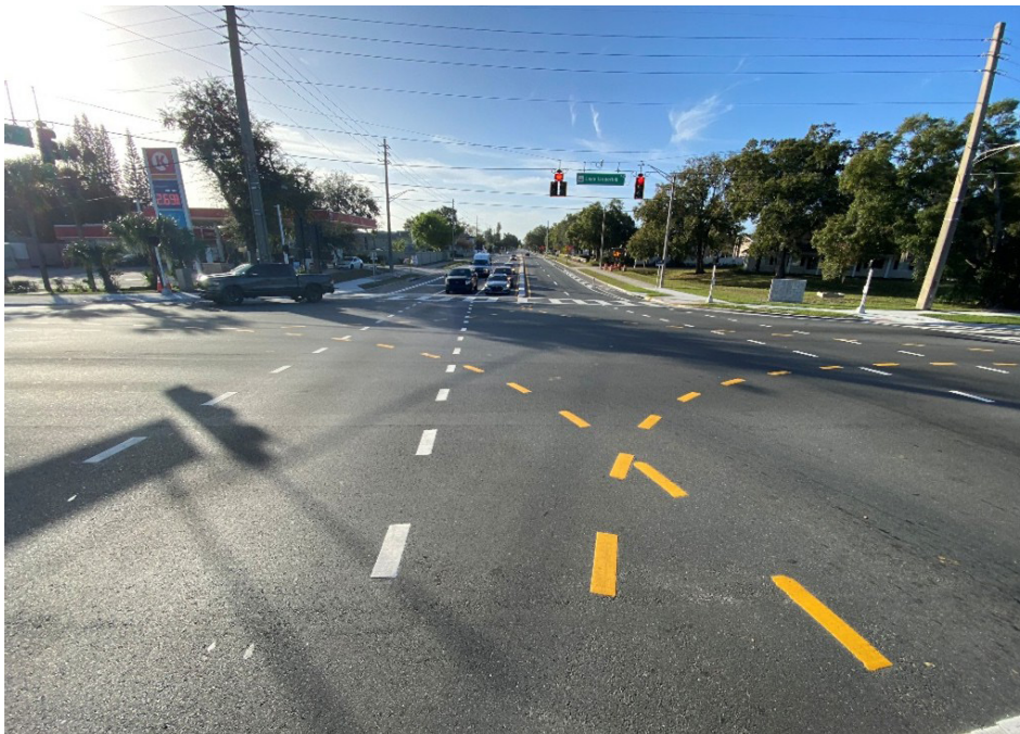
Figure 81: Intersection Dotted Guide Lines on Crystal Lake Road
