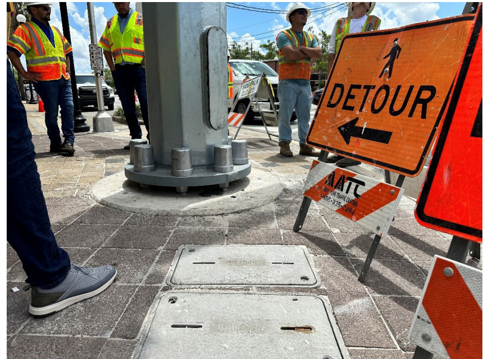
Figure 100: Example of a New Mast Arm and Foundation during Construction
