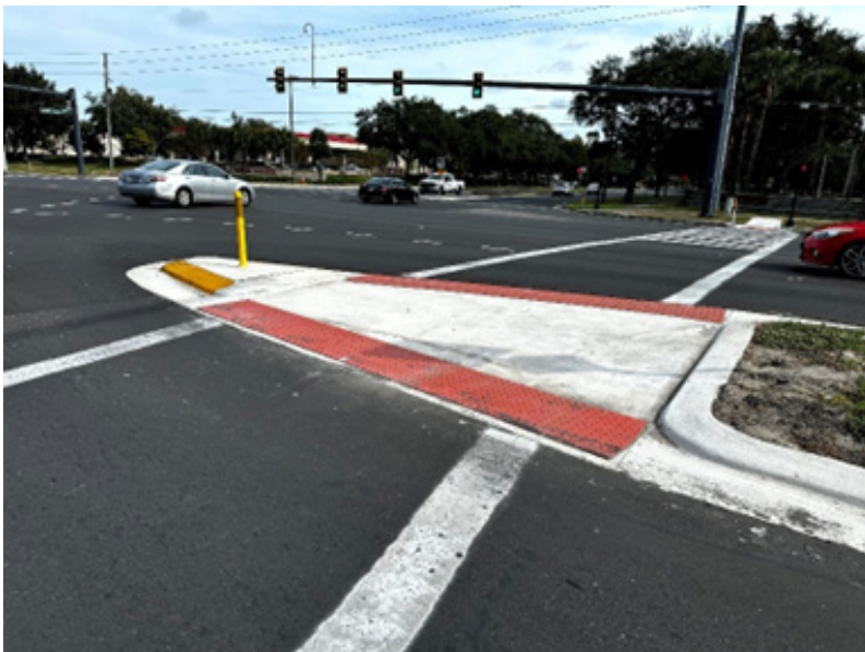
Figure 110: New Signalized Crosswalk and Concrete Refuge on SR 434
