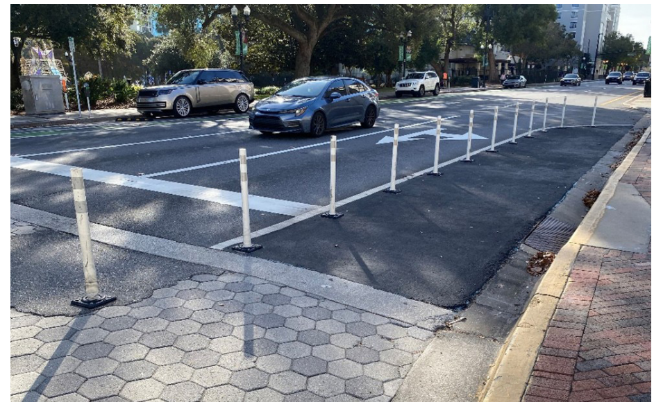
Figure 99: Photo of Curb Extension (Bulb-Out) on Rosalind Avenue
