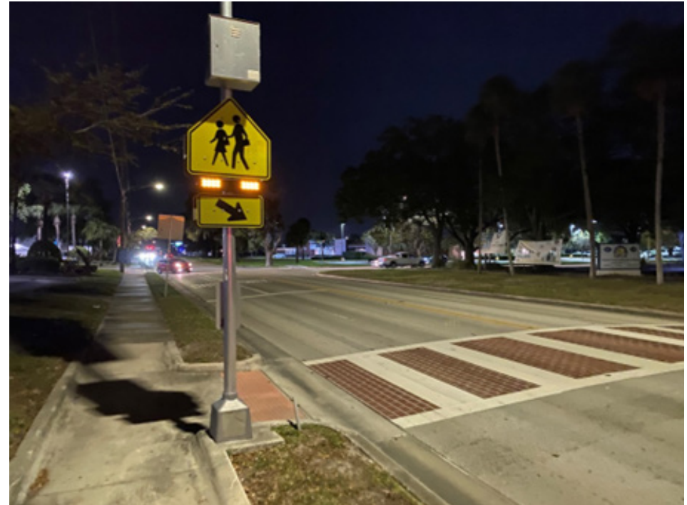
Figure 105: Rectangular Rapid Flashing Beacon Assembly on Primrose Drive
