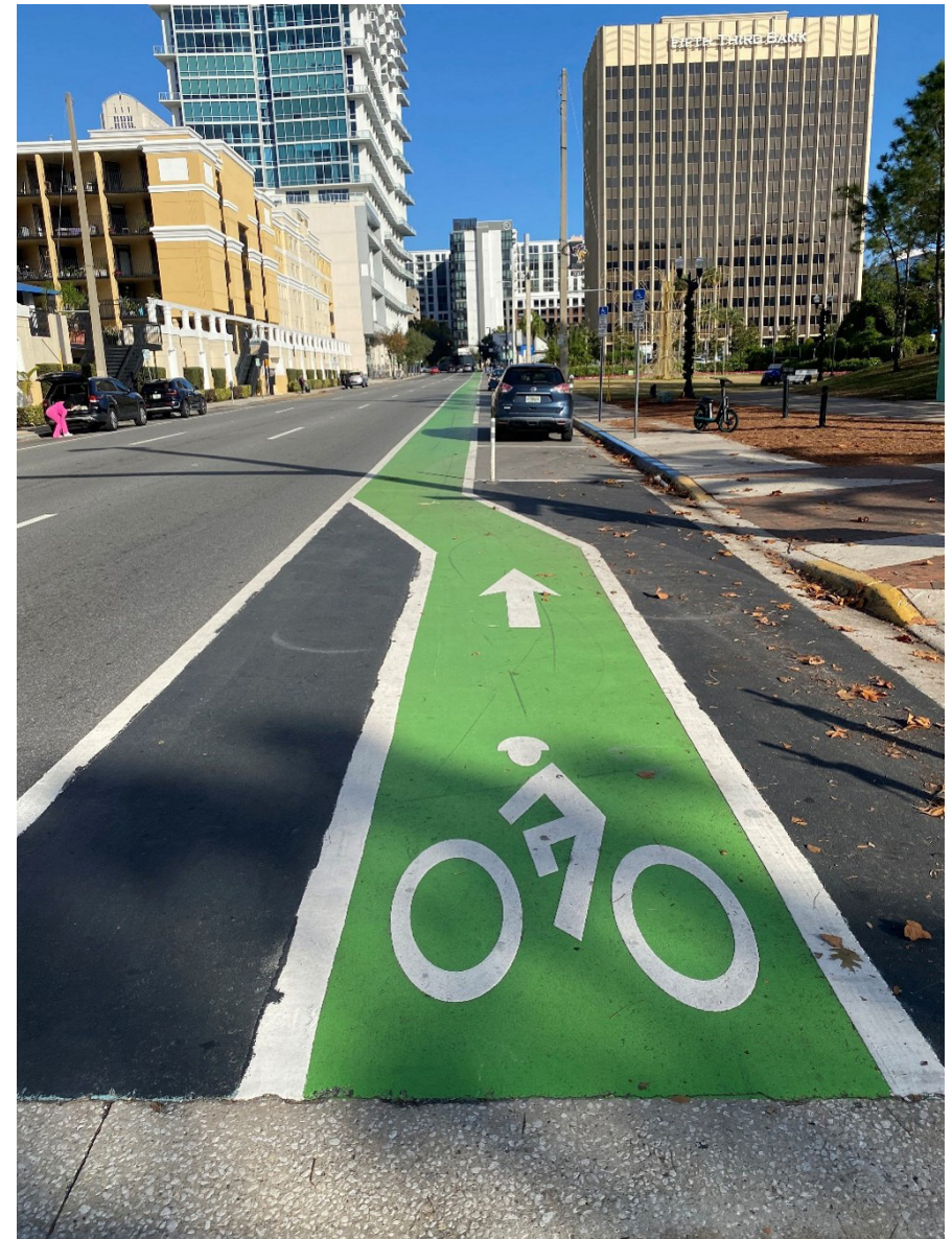
Figure 93: Solid Green-Colored Bicycle Pavement Markings on Rosalind Avenue
