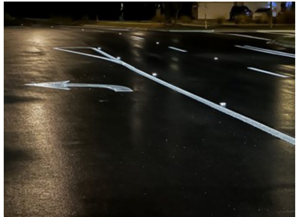
Figure 95: Photo of Raised Pavement Markers (RPMs) during Wet Nighttime Conditions
