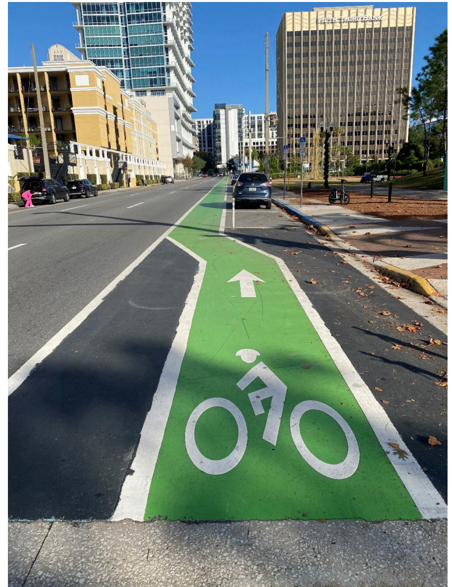
Figure 79: Solid Green-Colored Bicycle Pavement Markings on Rosalind Avenue
