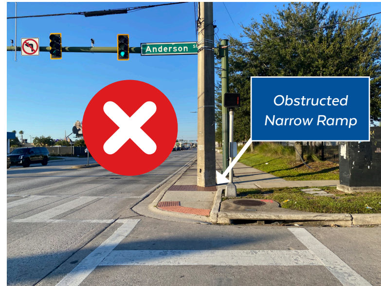
Figure 59: Obstructed and Unobstructed Curb Ramps on Orange Blossom Trail
