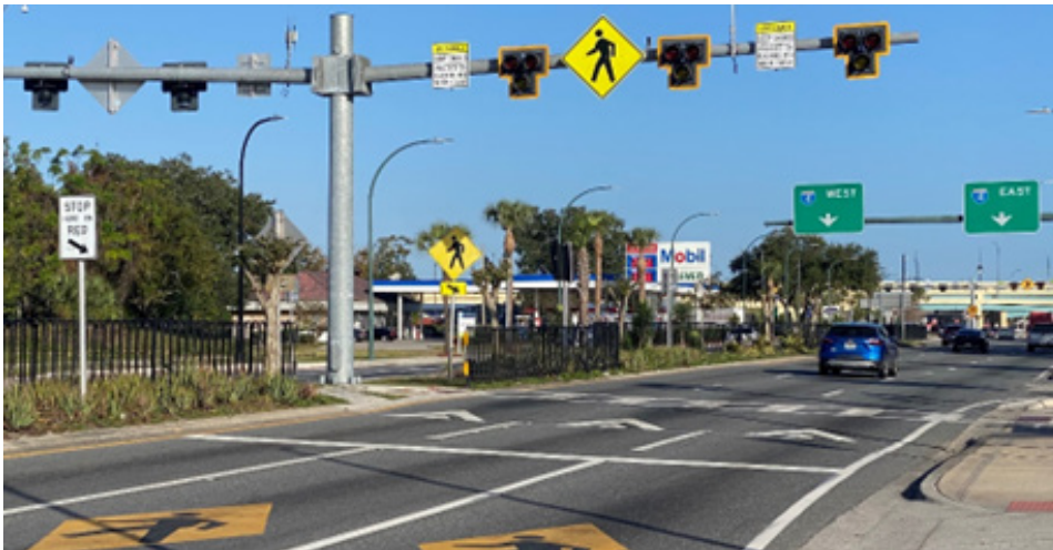
Figure 98: PHB with Raised Crosswalk on Orange Blossom Trail
