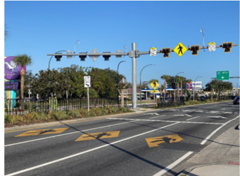
Figure 93: Functionality of the Pedestrian Hybrid Beacon Sequence
