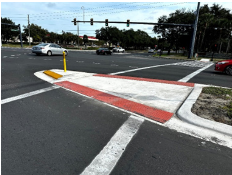
Figure 94: New Signalized Crosswalk and Concrete Refuge on SR 434
