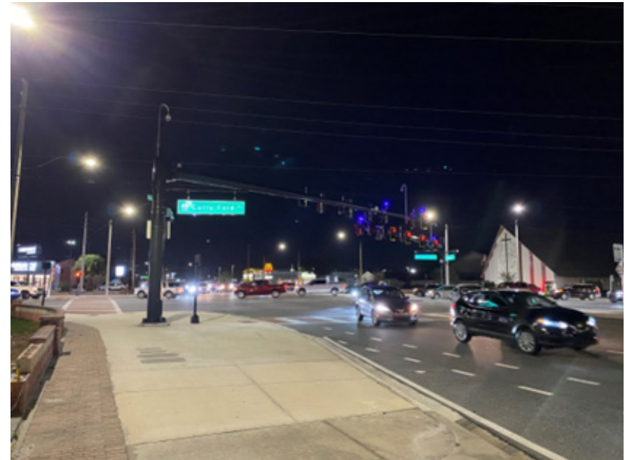
Figure 95: Intersection Lighting Enhancements on Curry Ford Road
