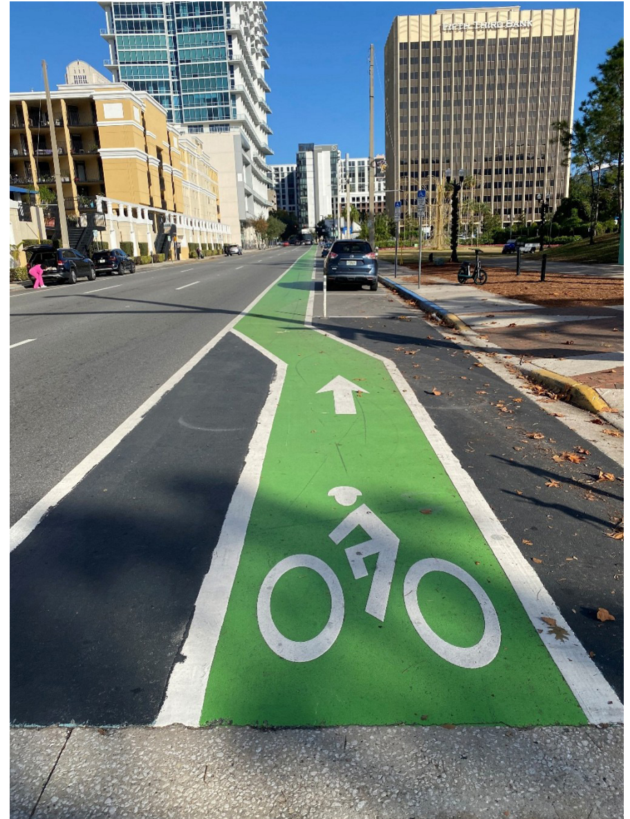
Figure 77: Solid Green-Colored Bicycle Pavement Markings on Rosalind Avenue
