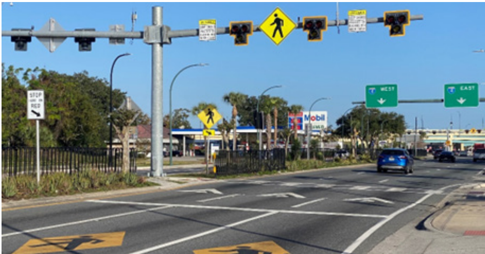
Figure 96: PHB with Raised Crosswalk on Orange Blossom Trail
