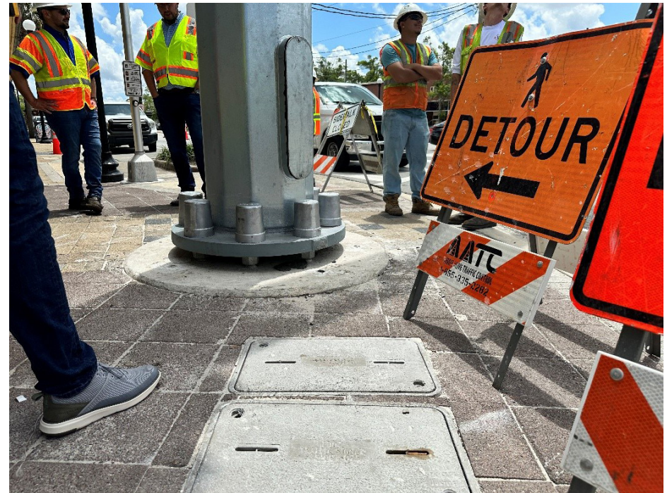
Figure 84: Example of a New Mast Arm and Foundation during Construction
