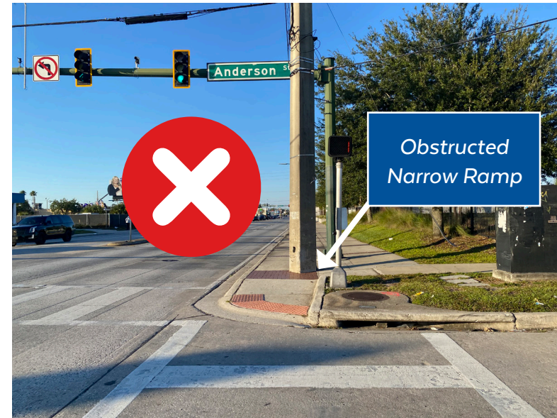
Figure 57: Obstructed and Unobstructed Curb Ramps on Orange Blossom Trail
