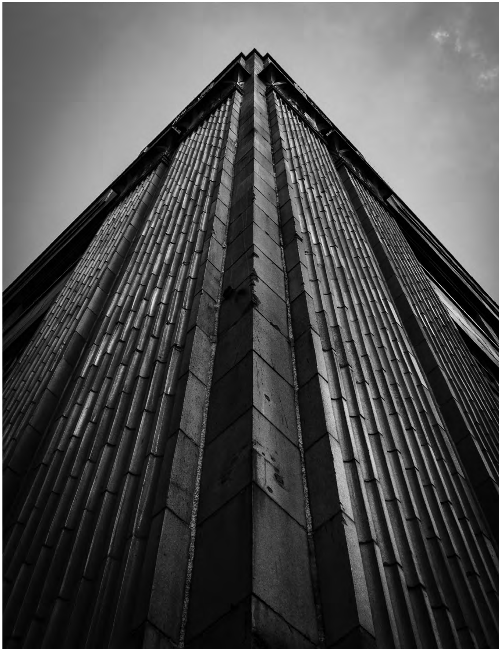
190 S. Orange Avenue, Downtown Historic District
