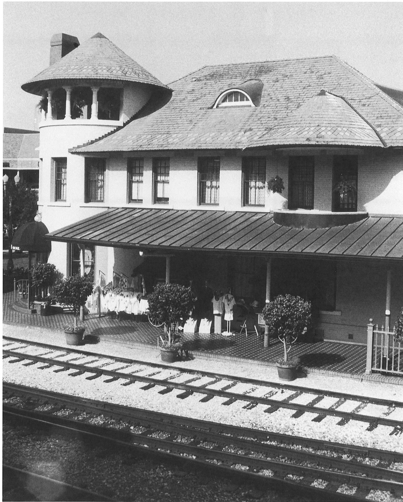
South Florida Railroad Depot • 76 West Church Street • 1889 • Photograph by Nancy Granger
