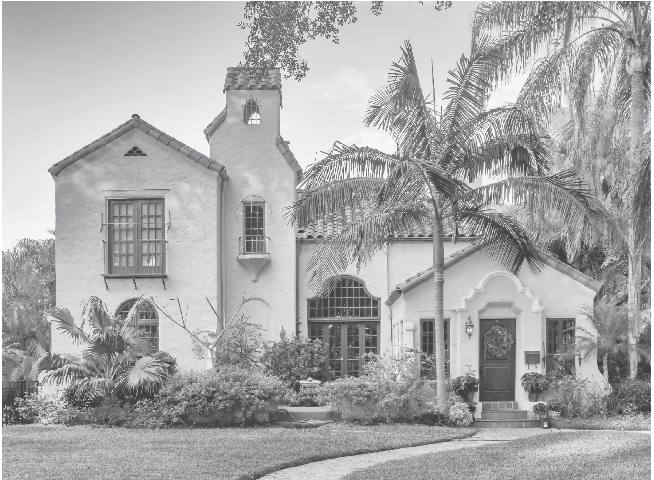
205 East Copeland Drive • Photo by Bob Egleston
