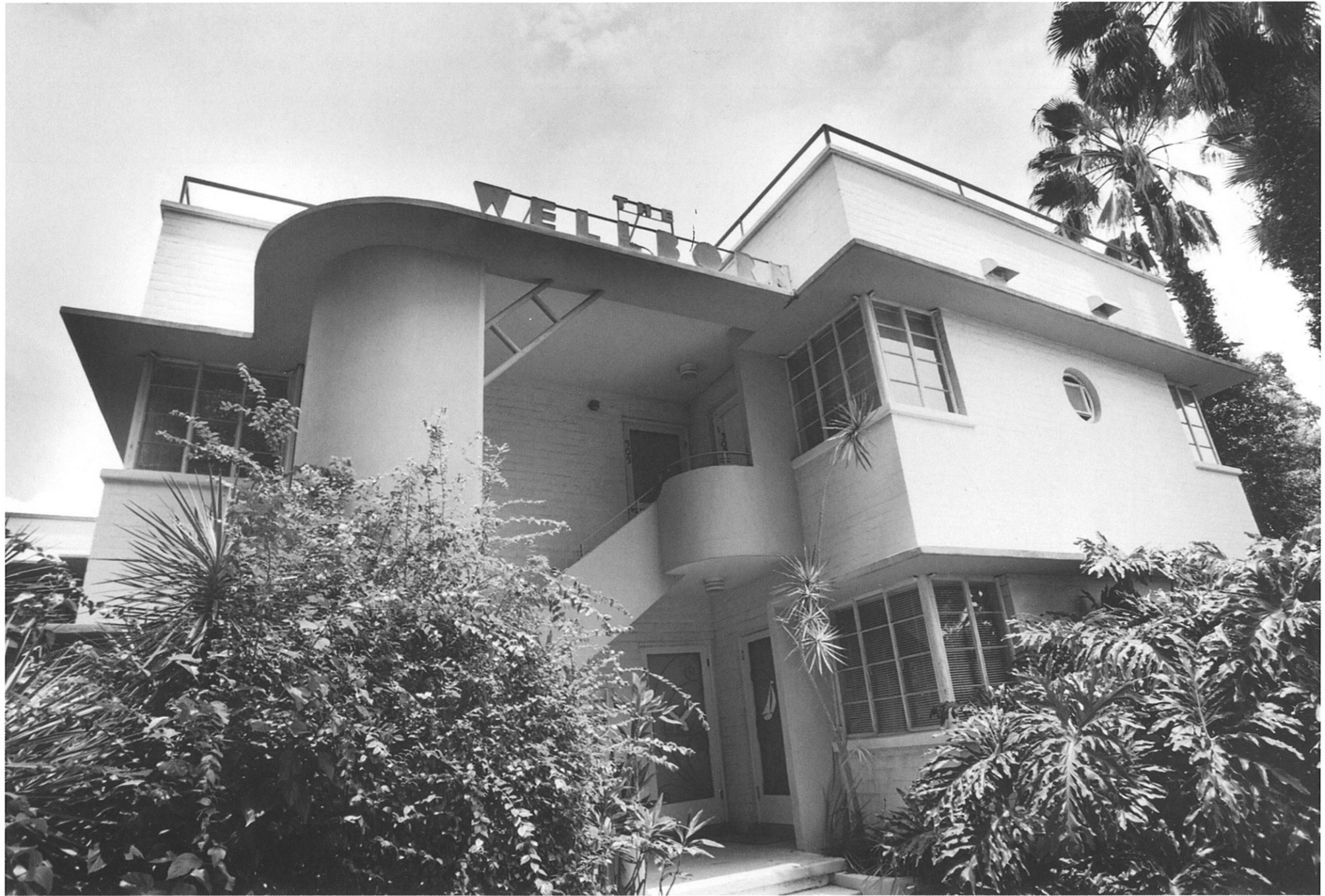
203 North Lucerne Circle East • Wellborn Apartments • 1946 • Photograph by Rose Jerome
