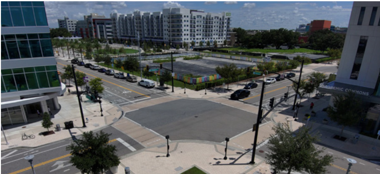
Figure 17: Median refuge islands reduce pedestrian exposure when crossing roadways and can be designed with mountable curbs to support fire department access.
