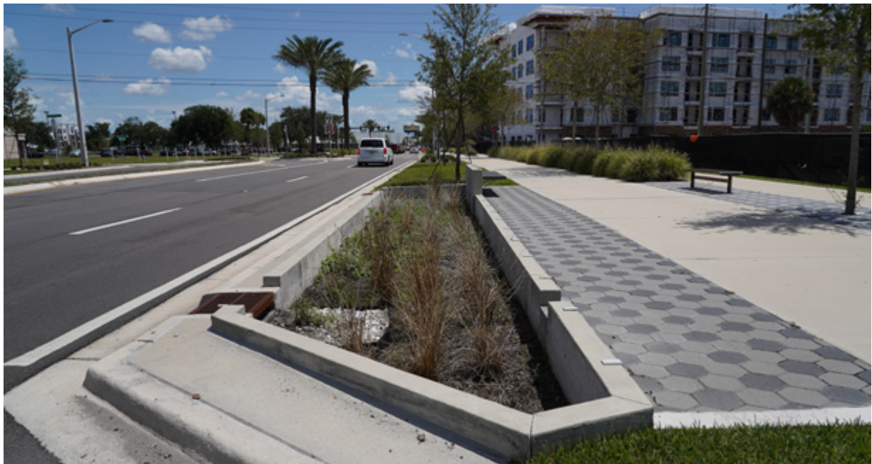
Figure 14: Curb extension create tighter corners and therefore reduces turning speeds of vehicles.
