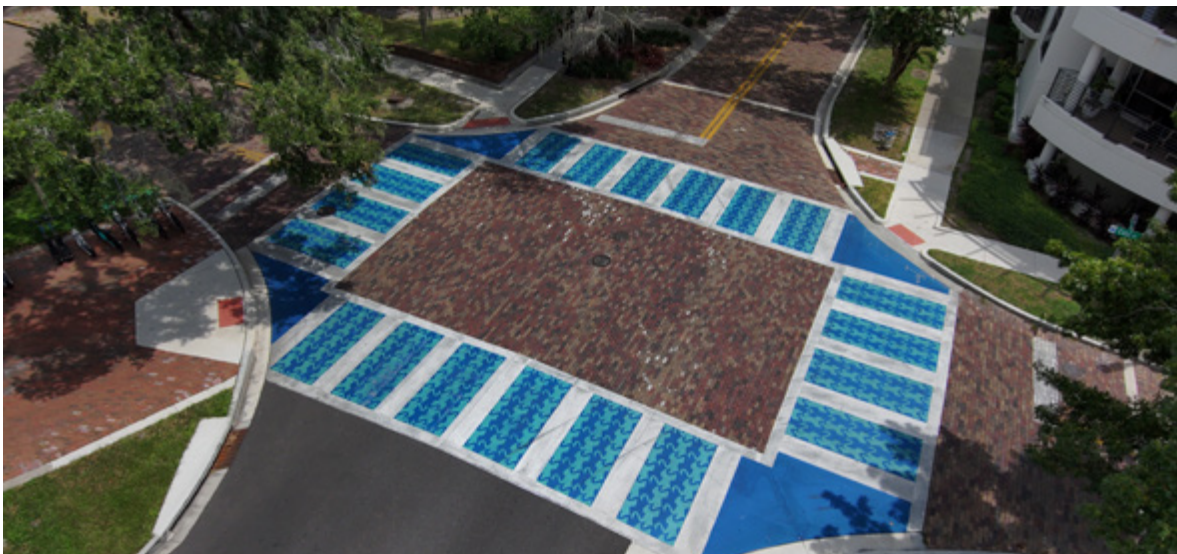
Figure 18: Raised intersections slow down regular drivers while providing adequate emergency vehicle access.
