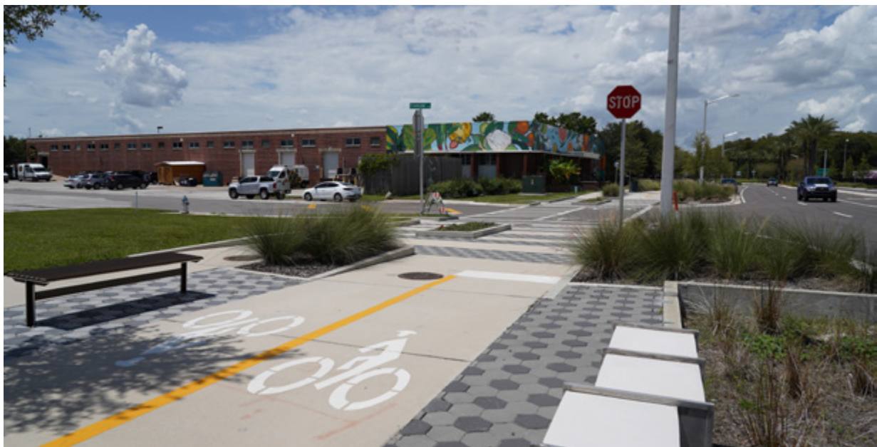
Figure 13: Bulb-outs create shorter crosswalk distance for pedestrians.
