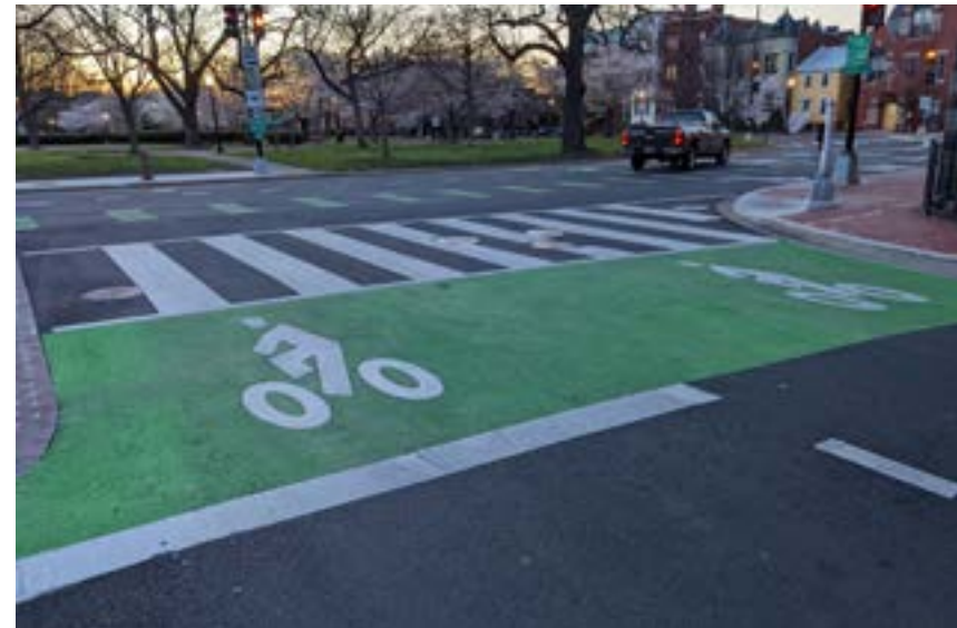
Washington, D.C. (Kittelson & Associates, Inc.)
