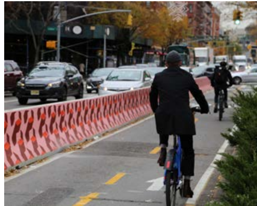
New York, NY. Source: NYC Department of Transportation
