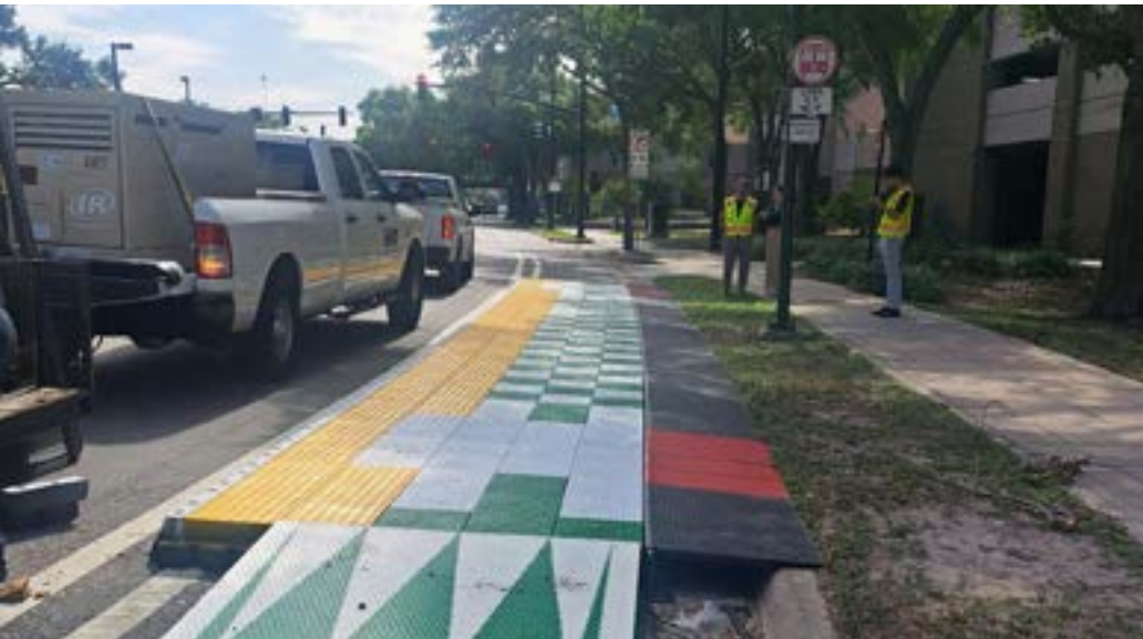
Amelia Street Bike Lane Bus Boarding Platform (City of Orlando)
