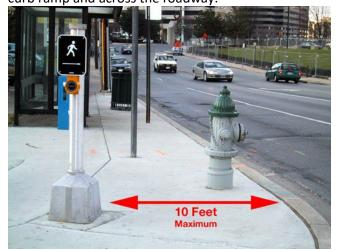
While the PROWAG Guidelines do not specifically address this issue, the U.S. Access Board Guidelines Section X02.5.1.3E states that the push button shall be mounted no further than 5 feet from the extension of the crosswalk lines, and within 10 feet of the curb line, unless the curb ramp is longer than 10 feet.
