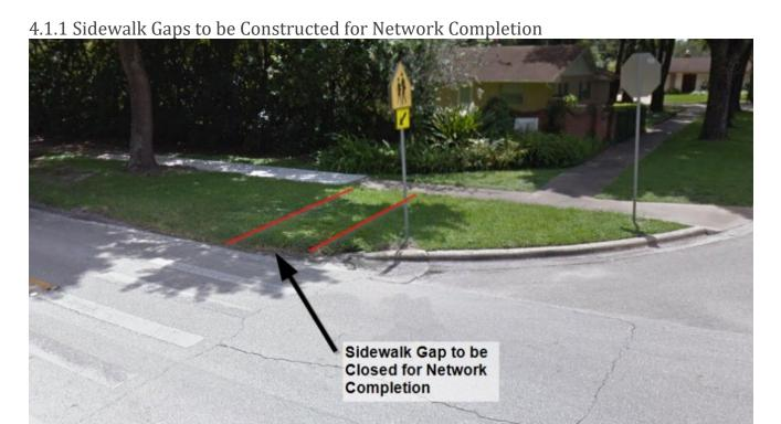
Sidewalk gaps are discontinuities in the pedestrian access route where the existing pedestrian access route ends abruptly or does not permit pedestrian access to the roadway as part of a pedestrian street crossing.
