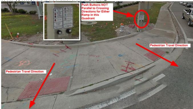
While the PROWAG Guidelines do not address pedestrian detector pushbutton orientation directly, the Guidelines incorporate the MUTCD Section 4E by reference, the 2009 Edition of the MUTCD Section 4E.08.04F calls for a pedestrian detector pushbutton orientation with "the face of the pushbutton parallel to the crosswalk to be used;".
