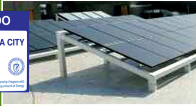
Four-kilowatt PV array at Edgewater High School
