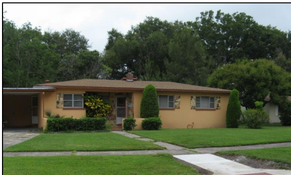
Figure 18: Examples of T-3 development. These are existing homes.
