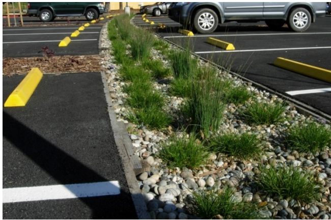
Figure 37 – Parking lot with bioswale
