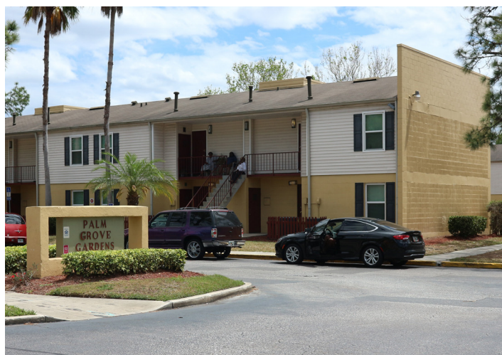
Figure 14: Palm Grove Gardens apartment complex.
