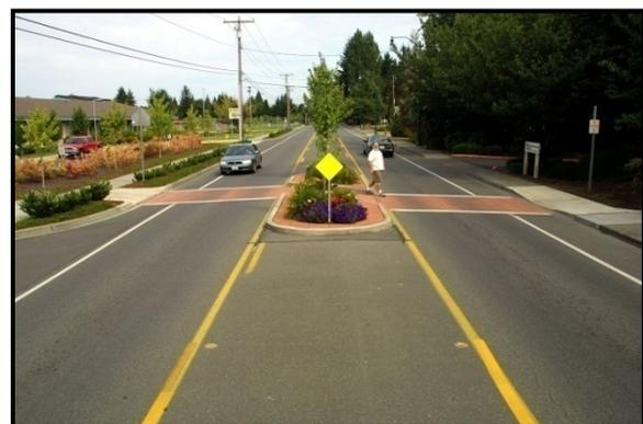
*Fig. 30* Crossings should use a variety of techniques, such as the off-set above, in order to enhance pedestrian safety.
