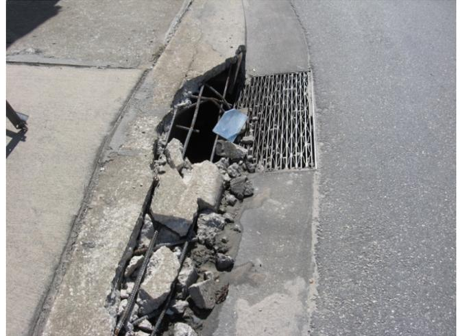
*Fig. 15.* Damaged curbs need maintenance.
