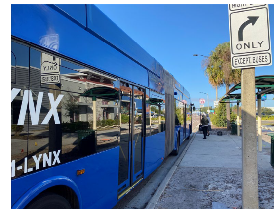
Bus bay too short for articulated bus.
