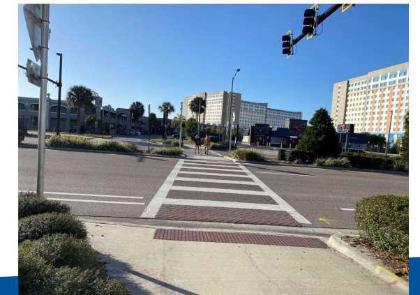
Midblock pedestrian signalized crossing.
