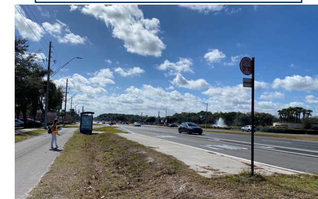
Bus bay missing sidewalk connection.
