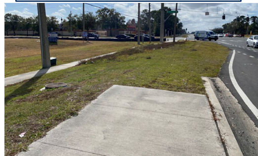
Missing connection to sidewalk from bus bay.
