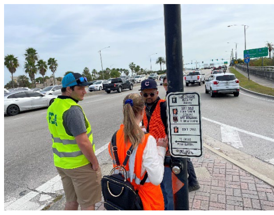
Mislabeled pedestrian crossing push-button signage.
